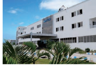
Rudrapur Plant (Green Building)
